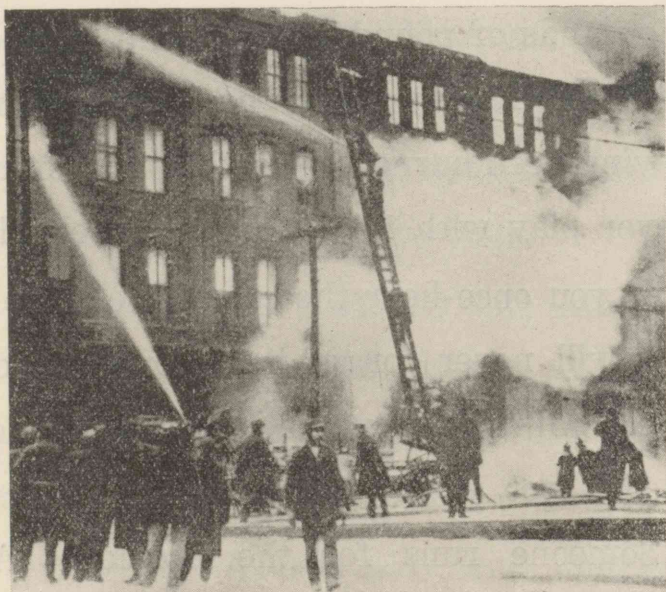
MODERN FIRE APPARATUS IN ACTION.
